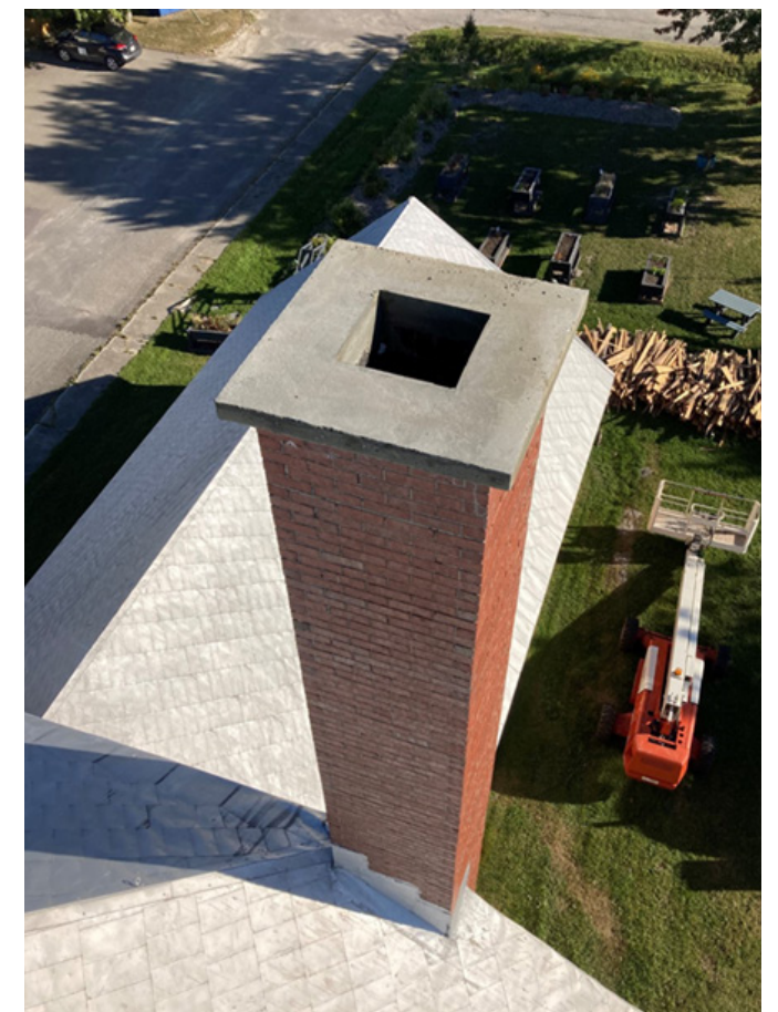
The newly renovated chimneys of the Saint-David de Sully church, in Quebec. Photos by Steve Thériault.
